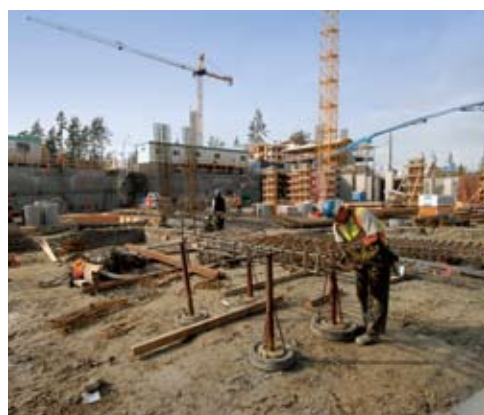
Excavation and foundation work is well underway
